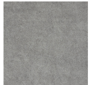
Exterior Stairs Concrete
